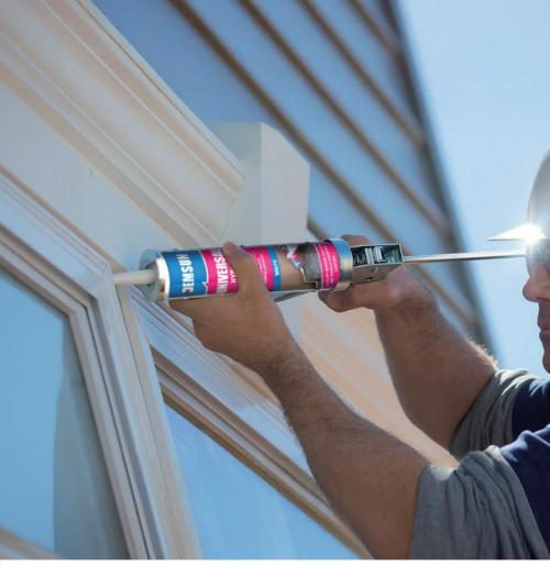
Highly thixotropic: Suitable for horizontal and vertical joints. Eco-friendly, free from isocyanate, solvent, acids and halogens.
